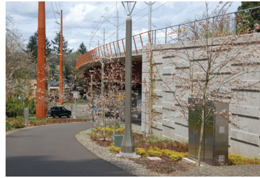
A filled guideway structure with enhanced architectural treatments and a multiuse path in a neighbourhood setting
