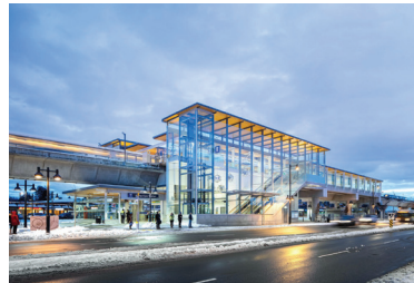
A public, multiuse path sharing the underside of an elevated LRT guideway
