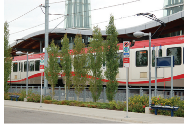
Station public realm enhancements
