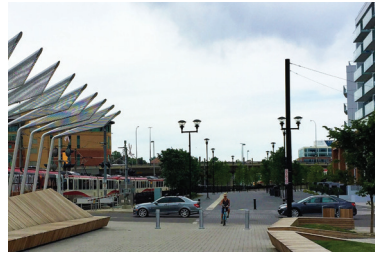
Multiuse path, lighting and landscaping with a separated right-of-way LRT
