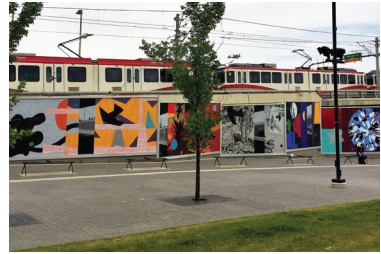
A filled guideway structure with public art mural treatments and a multiuse path in a redeveloped area
