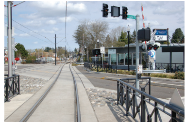
Enhanced LRT design treatment in an exclusive right-of-way within an historic community centre
