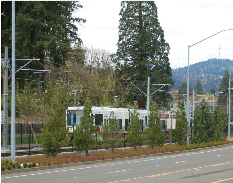
Enhanced landscaping, fencing and lighting in an exclusive right-of-way with an adjacent arterial
