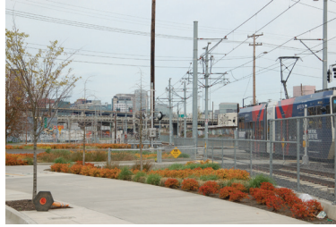
LRT crossing with enhanced public realm in an industrial area
