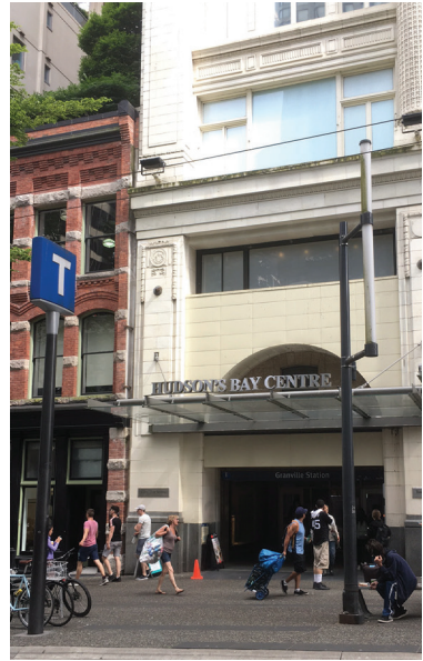
Station headhouse incorporated into commercial/retail development; at-grade public realm enhancements at station block.
