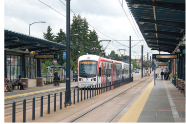
Station platforms in a low-floor system
