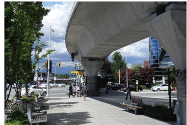
Enhanced pedestrian public realm under a rail guideway
